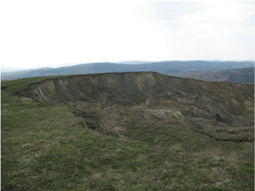
Fig. 10.4 Waste dump affected by a recent deep-seated landslide, Mateești (Getic Subcarpathians) (Photo: Marta Jurcescu)
